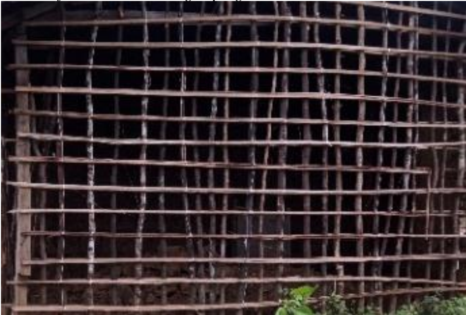
Sticks installed for walls in Odioabidi community (Source: researcher 2024)
